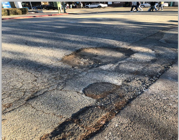
Potholes and Broken Asphalt on an Oakland Street
