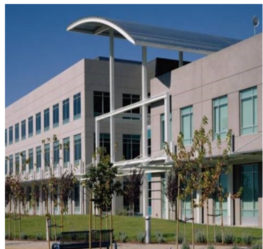
The Zhone Building, Oakland
