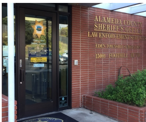
Eden Township Substation, San Leandro
